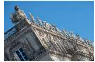
HchNS.I, Westfassade (Detail), DI018946, BSV
