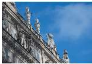
HchNS.I, Westfassade (Detail), DI018948, BSV
